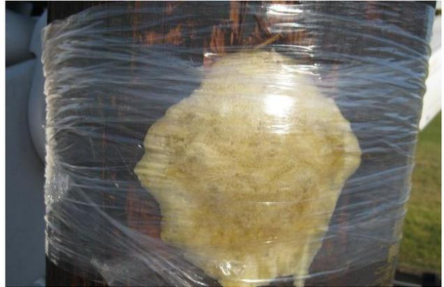
Woodpecker damage repaired with UPR™ Pole Repair
