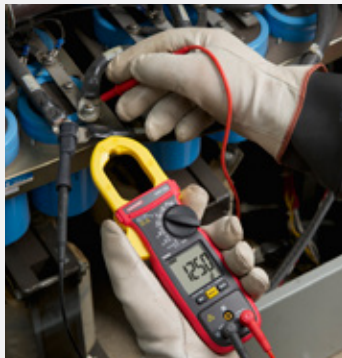
AMP-320 AC/DC Clamp Meter Electrical Motor Maintenance
