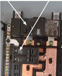
To activate standby power the utility main breaker must be in the "OFF" position to prevent dangerous feedback between the power sources.
