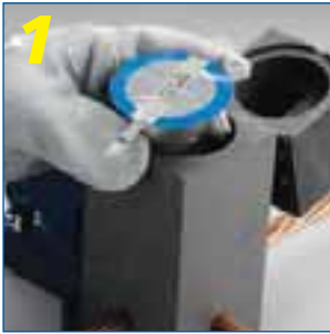
1 Insert CADWELD® PLUS package into mould
