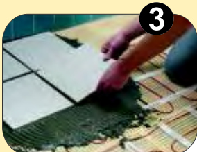
Install tiles/floor coverings
