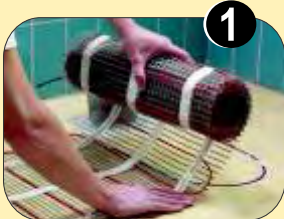
Unroll the self-adhesive mat onto the floor
