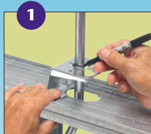
Place B44 on metal stud and mark EMT.
