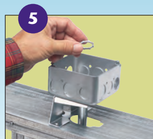
Install locknut on EMT fitting.
