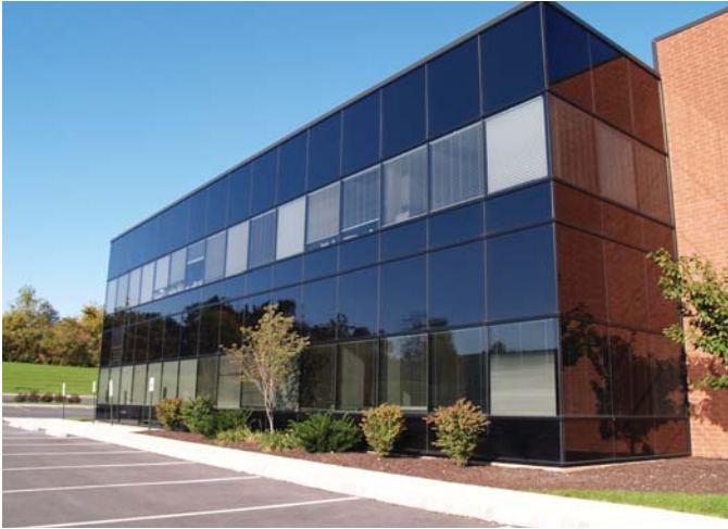
45 and 60 kW generators are ideal for most commercial applications including small office buildings, churches, retail centers, schools, and restaurants. Being light weight makes them appropriate for roof mounting.
